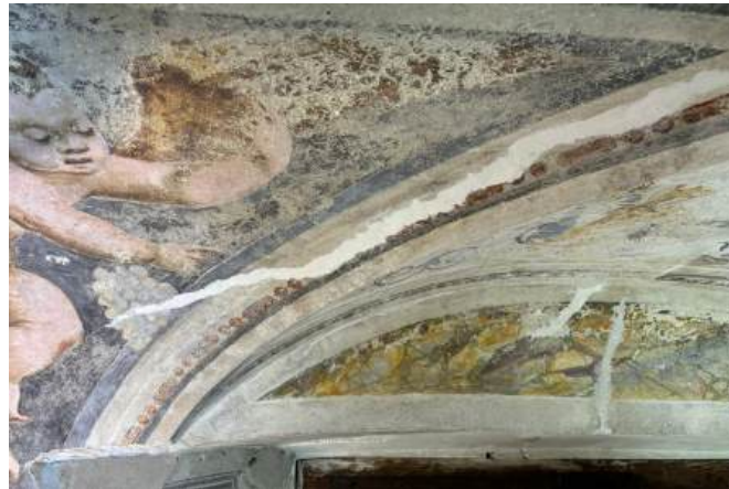
Fig 45 - Final Filling
