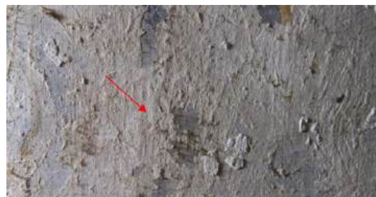
Fig 28 - Detail of second whitewash with fibers on lunettes, LNWI3
