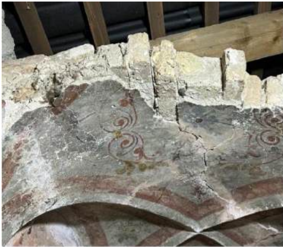
Fig 9 - View of the support of the vault staircase over the Vestibule
