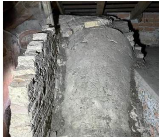
Fig. 10 - View of the vault of the staircase over the Vestibule
