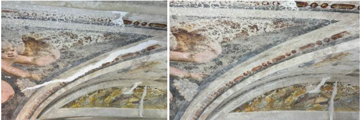
Fig 49 and 50 - Before and after application of Tratteggio
