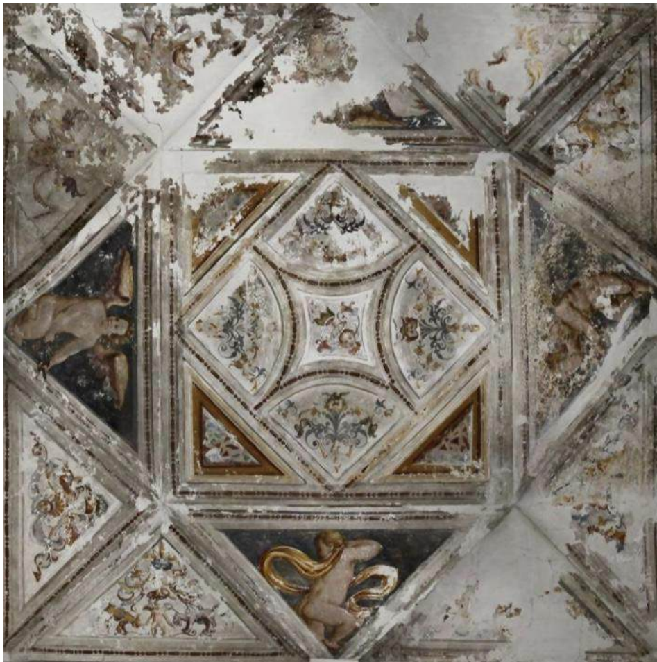
Fig 3 - The Vestibule Vault, before restoration intervention
