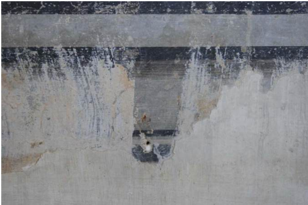
Fig 25 - Different layers of whitewash
