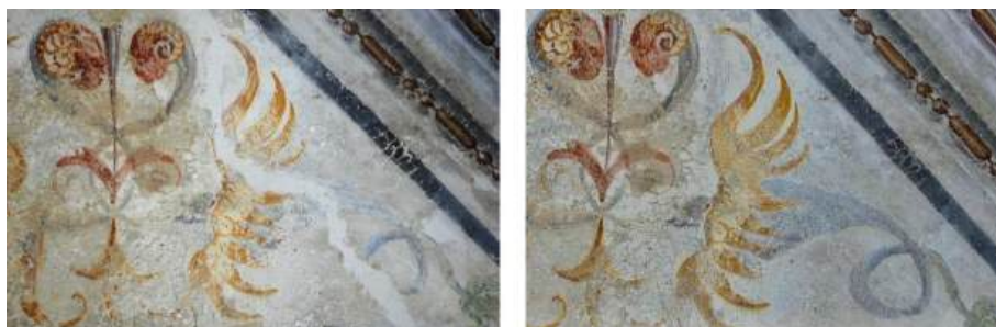
Fig 53 and 54 - Before and After Chromatic Integration of the ceiling
