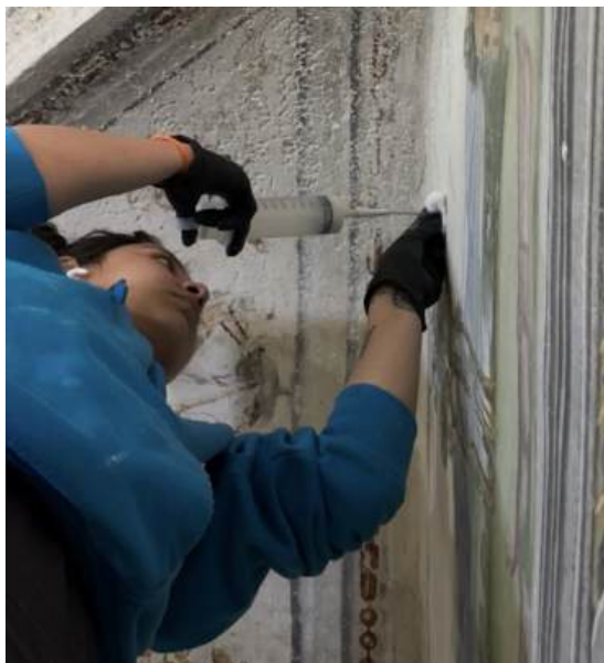
Fig 40 - Insertion of PLM-AL® (C.T.S.), prepared in a dilution of 100 g of powder in 100 g of demineralized water
