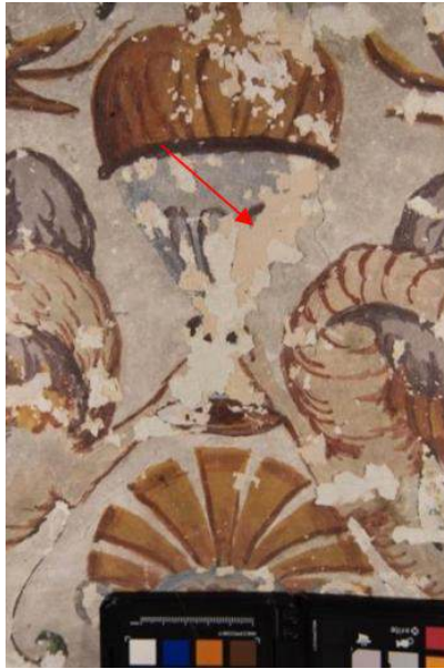
Fig 29 - Yellow whitewash layer on vault and lunettes, VNE1
