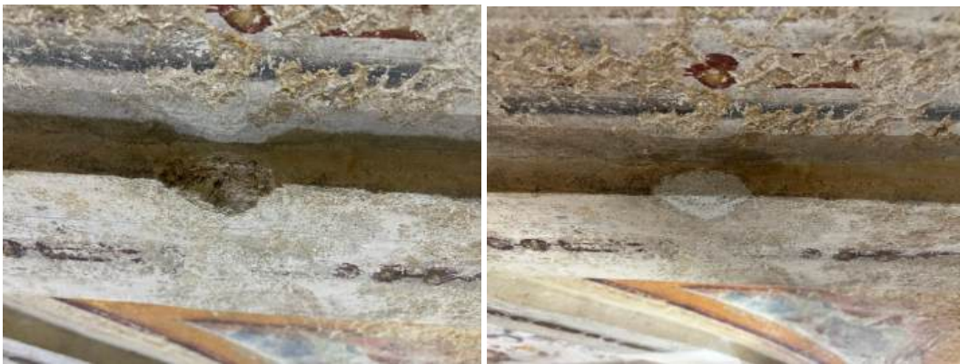
Fig 44 - Before and after reconstruction of a corner
