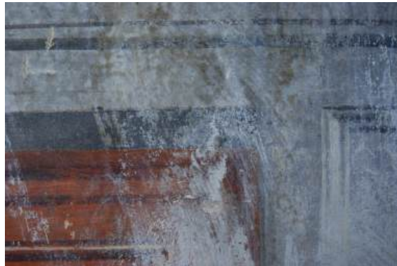
Fig 22 - Oldest Semi-transparent whitewash layer
