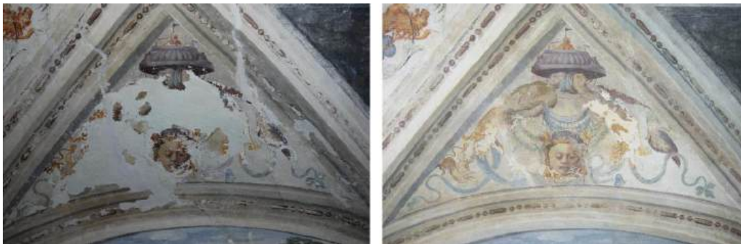
Fig 42 - Vault LNWI, before and after the mechanical descialbo performed with a scalpel.
