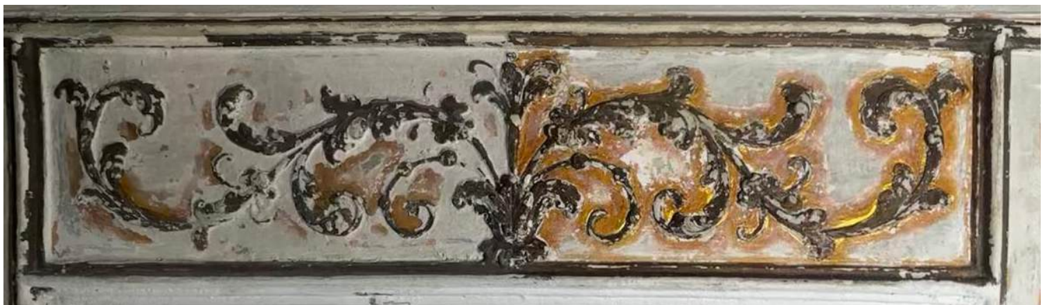
Fig.24 On the left is the unclean side in comparison to the cleaned side on the right
