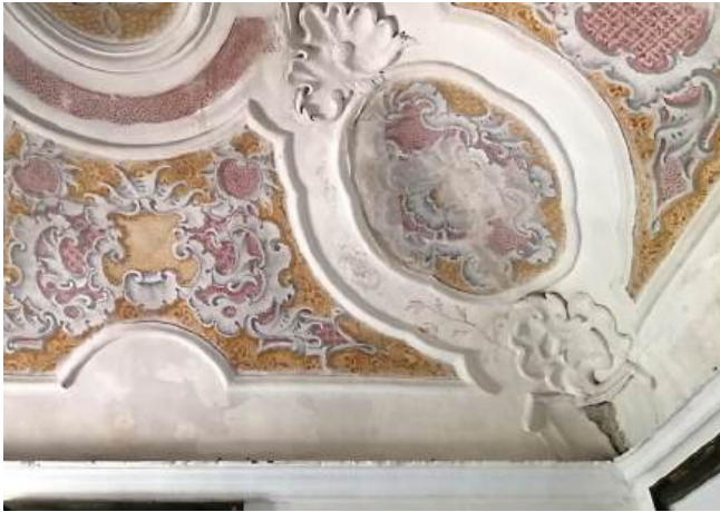
Fig.10. Baroque style painting with stucco frame in Room 3
