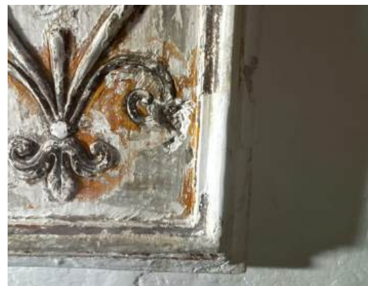
Fig.31 After filling the lacunae
