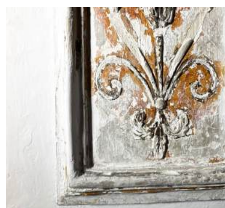
Fig.33 After filling the lacunae
