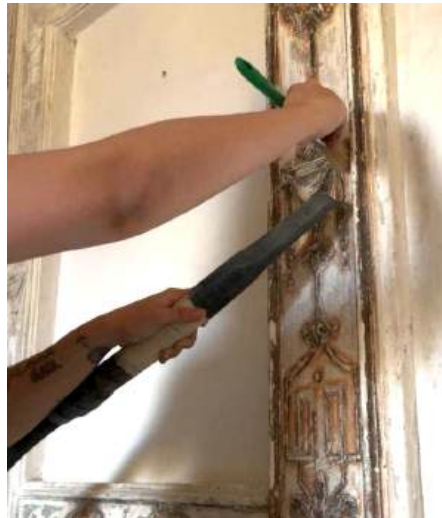
Fig.25 Cleaning dust particles with vacuum cleaner and a brush
