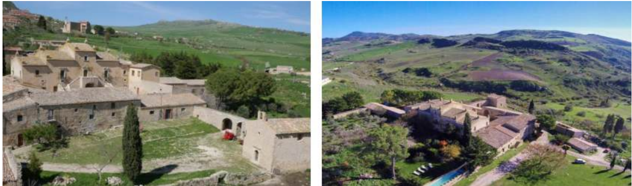
Fig.4. View of the second courtyard facade
