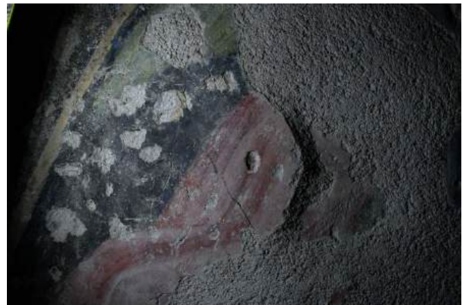
Fig.65,66. Cracks and fissures formed near existing fillings
