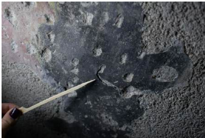
Fig.65,66. Cracks and fissures formed near existing fillings
