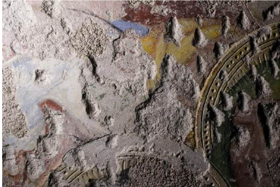
Losses that reveal the superimposition of different plaster layers
