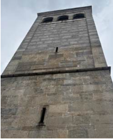
Fig.9. Evidence of different constructions on the bell tower
