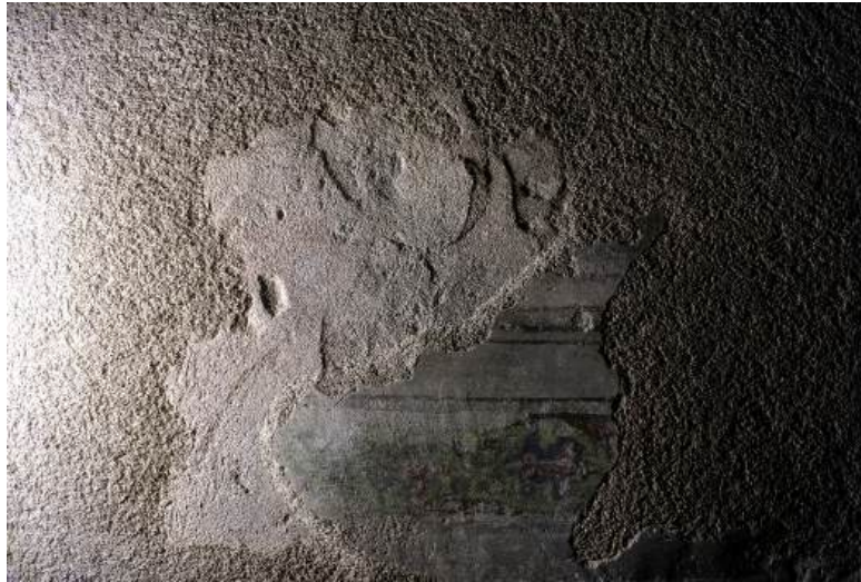
Base plaster (arriccio) with finishing plaster (intonachino), observed under raking light
