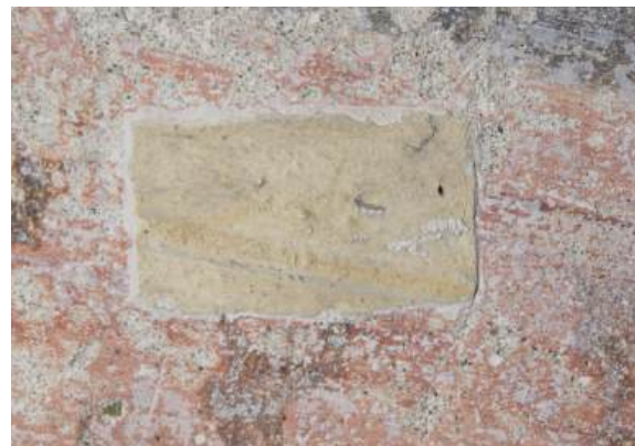
Fig.63. Evidence of Lime wash left behind by Gianola
