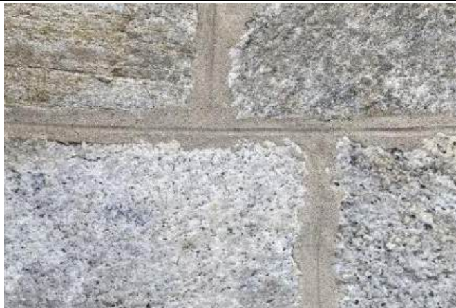
External masonry with visible tooled joints
