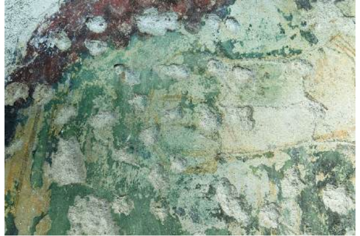
Abrasion of paint layer
