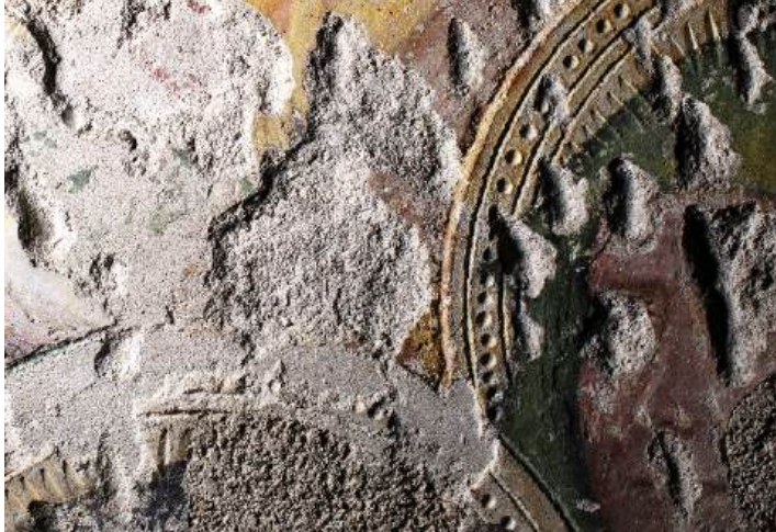
Abrasion of Intonaco
