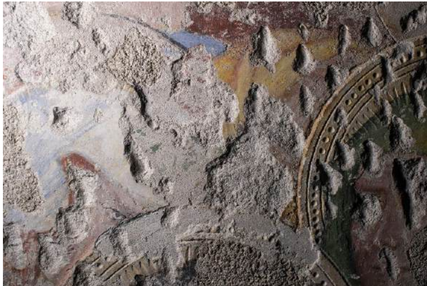
Area where a layer of pigment is visible beneath fallen plaster, possibly indicating a pentimento.
