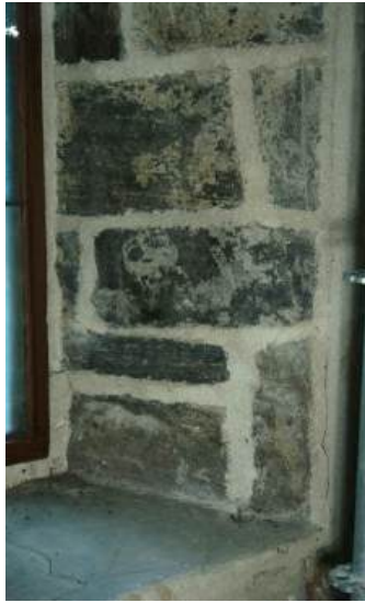
Masonry visible in the splay of a window
