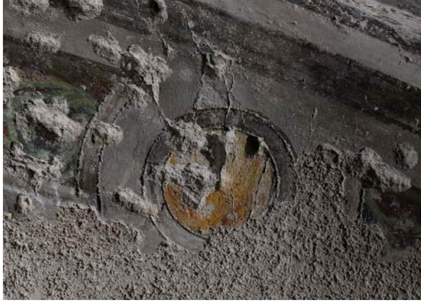
Direct incisions made with a compass, visible under raking light.
