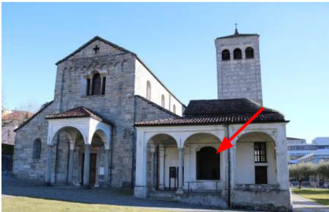
Fig. 7. The Chapel of the dead - Ossario
