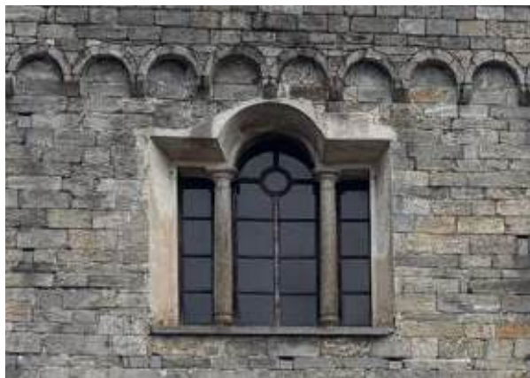
Fig.5. Serlian arched window replaced the original oculus
