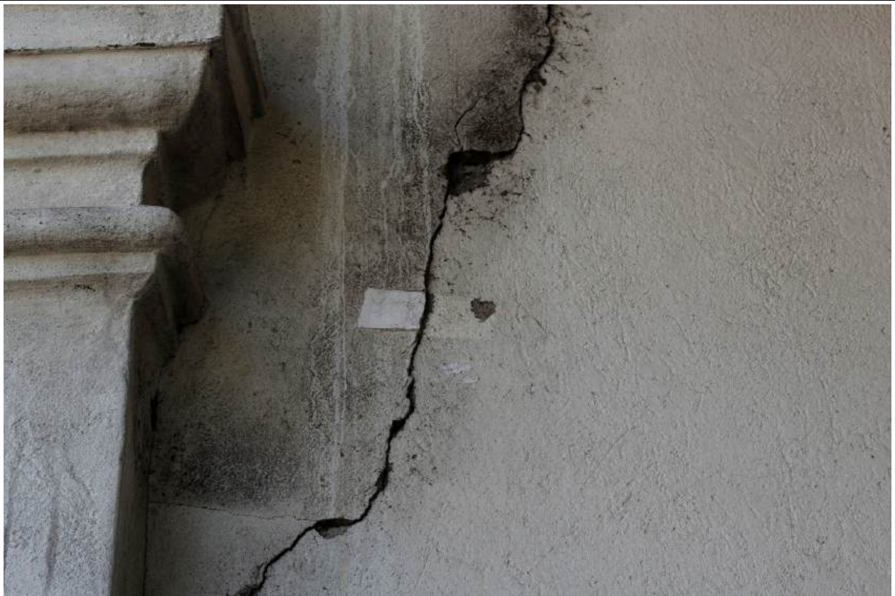
Activated Crack meter
