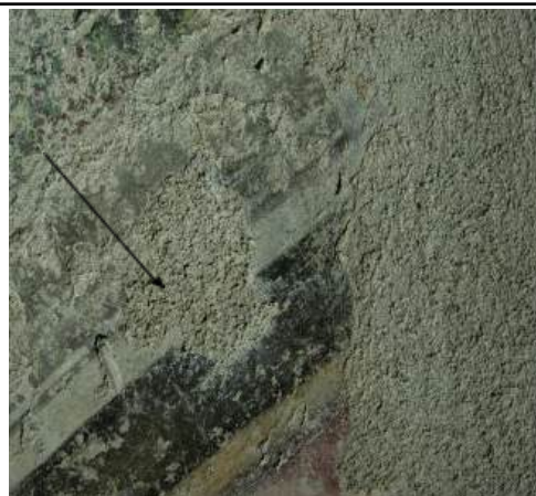
Stucco filling dating to the restoration work by Luigi Gianola
