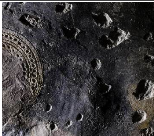
Joint between giornate with visible tool marks
