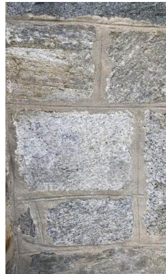
External masonry with visible tooled (or pointed) joints
